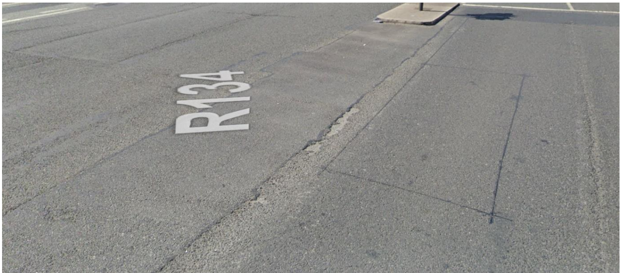
Figure 7-13: Moderate Road Pavement Condition at Nangor Road / Knockmitten Lane Junction with some ravelling around reinstatement works and joints ©2019 Google Maps
